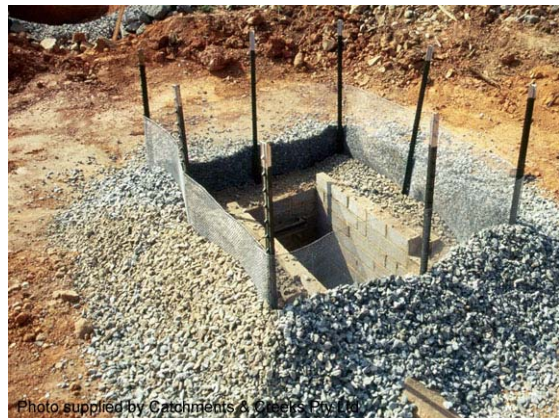
Photo 10 – Mesh & aggregate system
