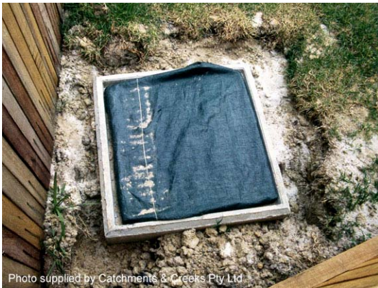
Photo 7 – Fabric wrap drop inlet protection
