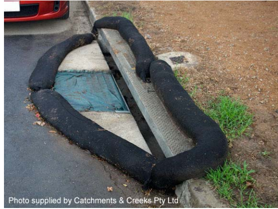
Photo 4 – Compost-filled filter sock
