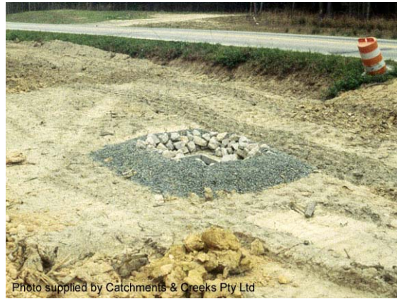
Photo 12 – Rock & aggregate system
