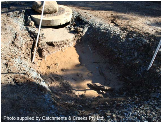
Photo 5 – Excavated drop inlet protection
