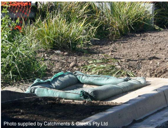
Photo 13 – Sandbags (filter sock)
