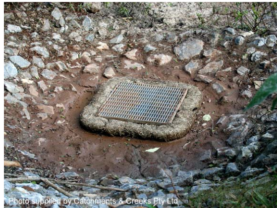
Photo 8 – Filter sock drop inlet protection
