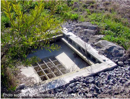
Photo 3 – Block & aggregate system
