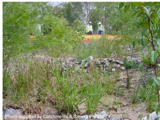
Photo 4 – Vegetated sediment trap (left) showing incorporated rock check dams
