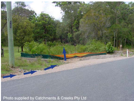
Photo 3 – Vegetated sediment trap placed at the outlet of a roadside table drain
