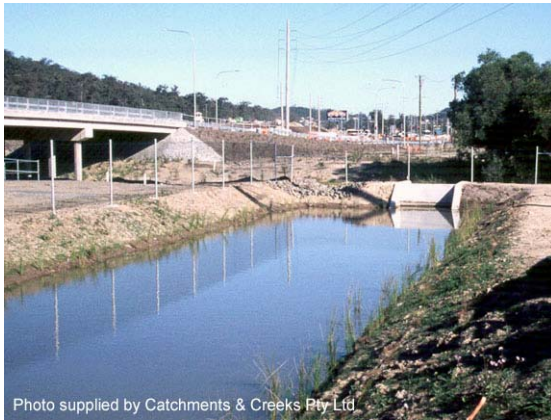
Photo 1 – Sediment basin (Type 1 system) Photo 2 – Rock filter dam (Type 2 system)
