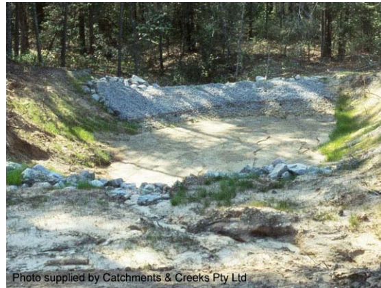
Photo 1 – Sediment basin (Type 1 system) Photo 2 – Rock filter dam (Type 2 system)
