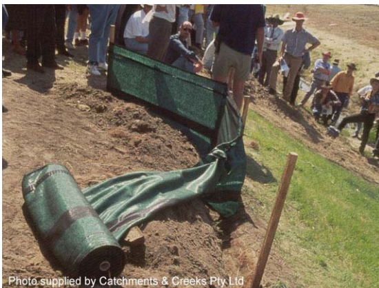
Photo 3 – Sediment fence (Type 3 system)
