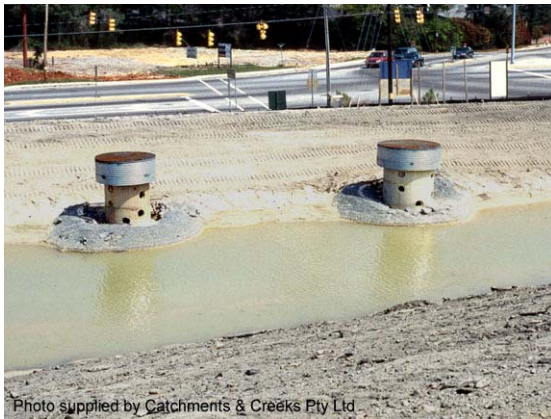
Photo 1 – Twin riser pipes in the process of being installed
