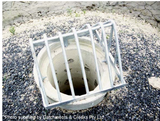
Photo 2 – Riser pipe with aggregate filter and trash screen
