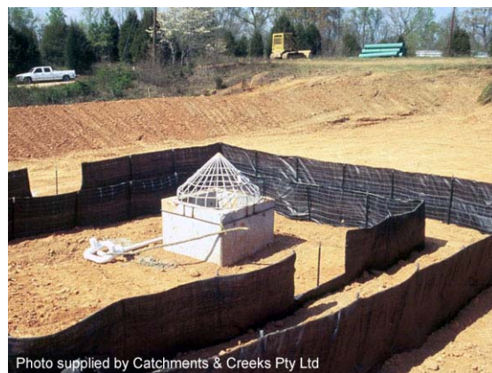
Photo 6 – Outlet chamber surrounding a flexible skimmer outlet device
