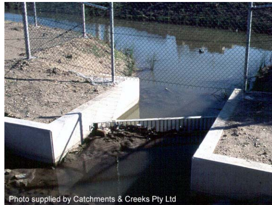
Photo 8 – Litter screen placed on inlet of permanent sediment basin
