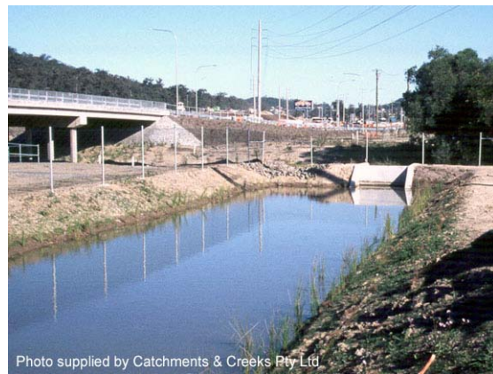
Photo 2 – Example of a 'wet' (Type F/D) sediment basin
