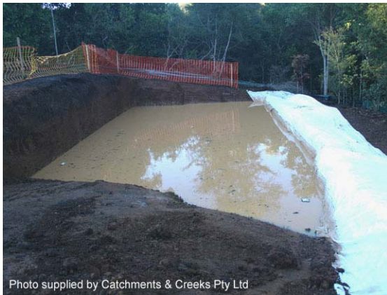
Photo 17 – Fully recessed basin with natural ground forming the spillway
