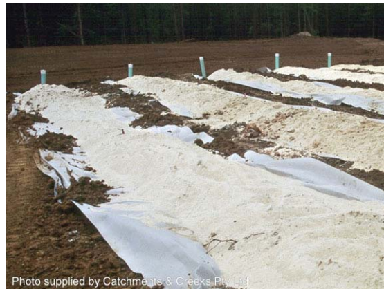
Photo 14 – Sand filter outlet system during installation
