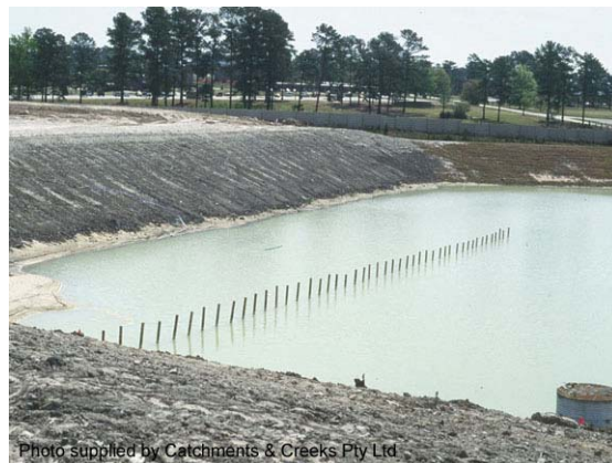
Photo 4 – Internal baffle extending the flow path between the basin inlet (left) and the basin outlet (right)
