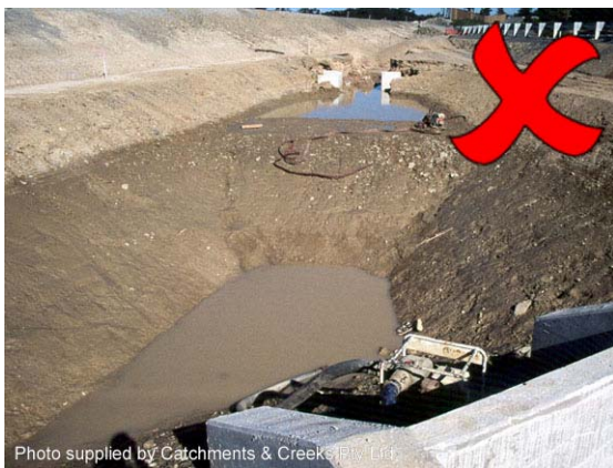
Photo 19 – De-watering pipe intake must not rest on the basin floor
