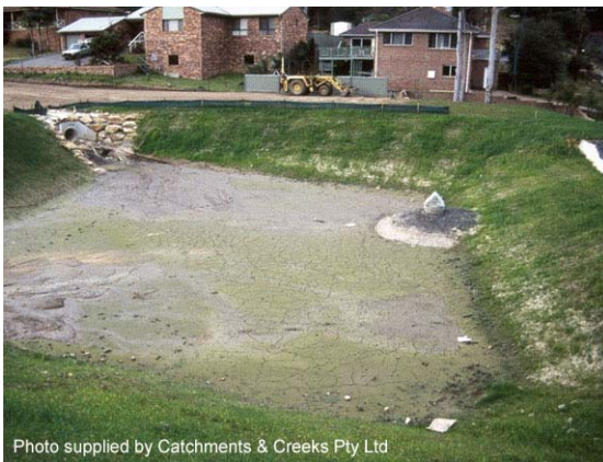
Photo 1 – Example of a 'dry' (Type C) sediment basin
