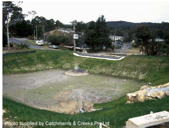
Photo 18 – Rock-lined spillway—note concrete sealing of the spillway crest
