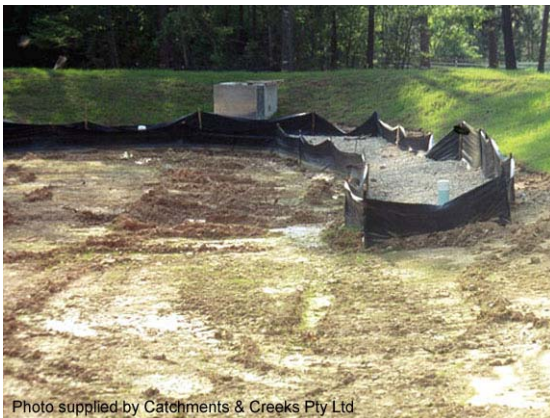
Photo 13 – Low-flow sand filter outlet system on a permanent sediment basin
