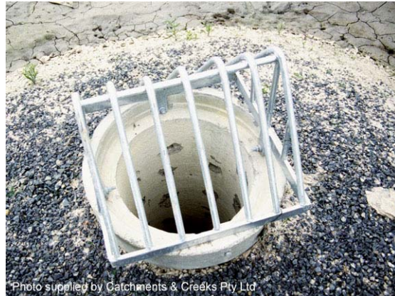
Photo 10 – Riser pipe with aggregate filter and trash screen
