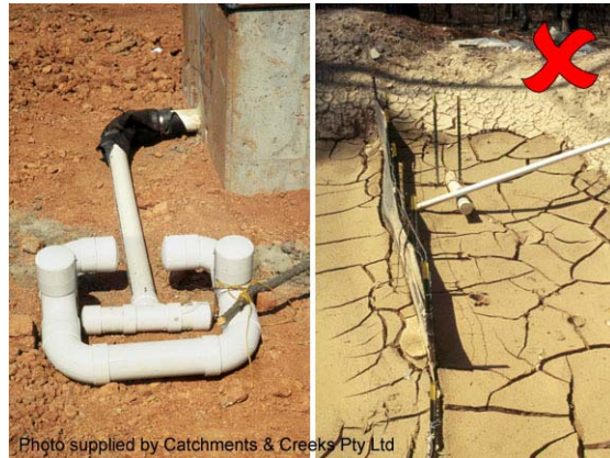
Photo 12 – Skimmer pipes must be protected from sediment build-up
