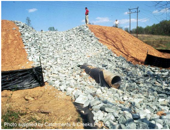
Photo 15 – Emergency spillway located within the fill embankment
