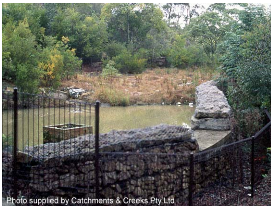
Photo 23 – Permanent sediment basin within residential estate
