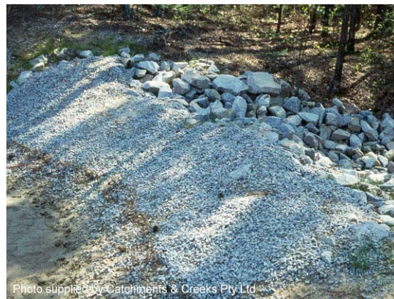
Photo 4 – Aggregate filter showing partial sediment blockage of lower area
