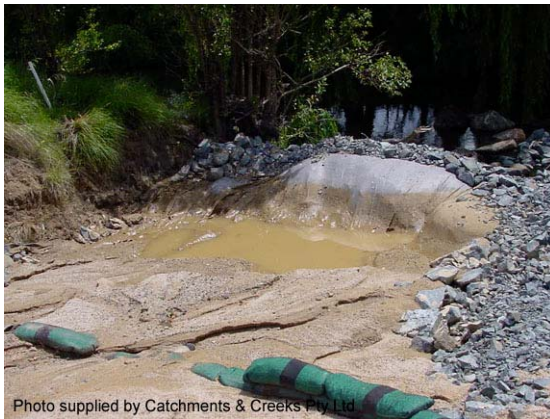
Photo 1 – Rock filter dam with geotextile filter
