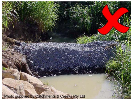
Photo 6 – The entire rock embankment should not be formed from small-diameter aggregate
