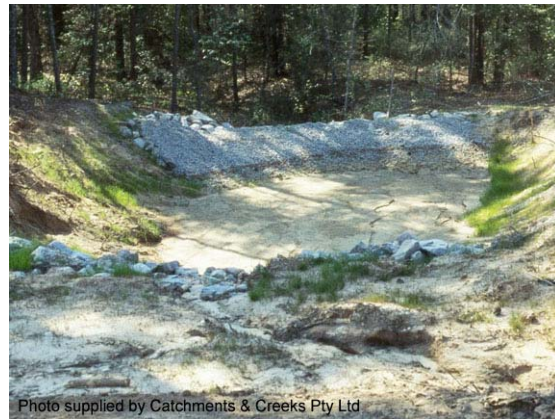
Photo 2 – Rock filter dam with aggregate filter
