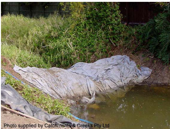
Photo 5 – Instream rock filter dam wrapped in filter cloth
