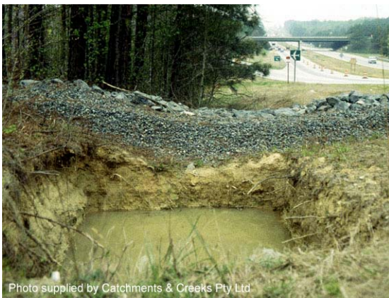
Photo 3 – Sediment collection pit upstream of rock filter dam
