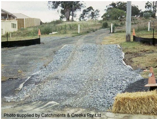
Photo 1 – Stabilised rock pad construction exit
