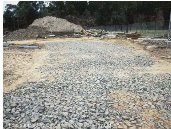
Photo 2 – Stabilised rock pad construction exit
