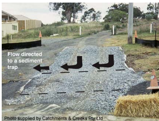
Photo 5 – Flow control berm
