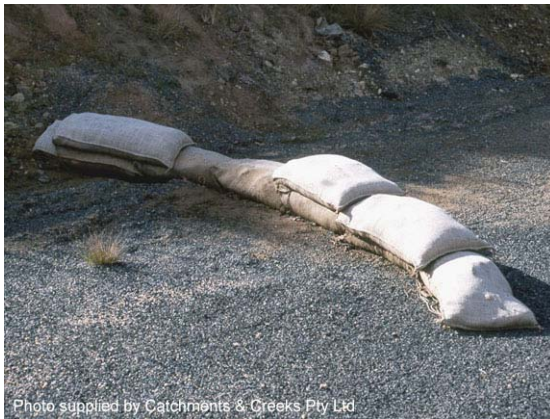
Photo 1 – Demonstration of sandbag placement to form a sediment collection dam with overflow spillway (centre)
