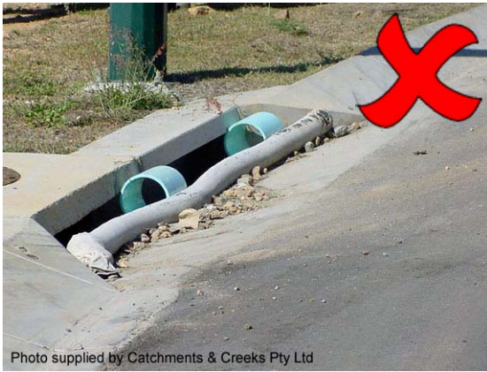
Photo 3 – Sediment trap must not be formed across the inlet of 'on-grade' kerb inlets (this type of sediment trap is only suitable for 'sag' inlets)
