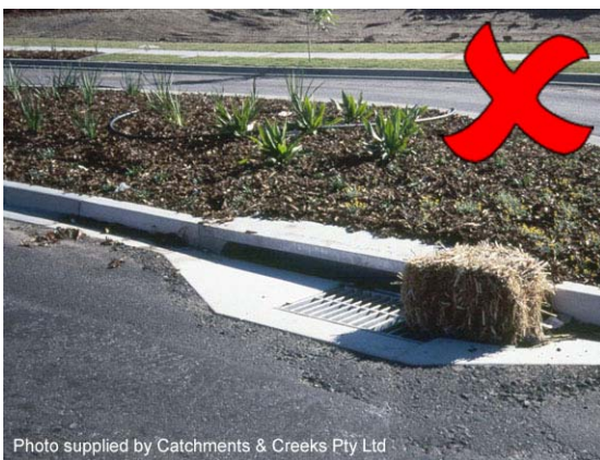
Photo 5 – Straw bales should not be placed on solid surfaces
