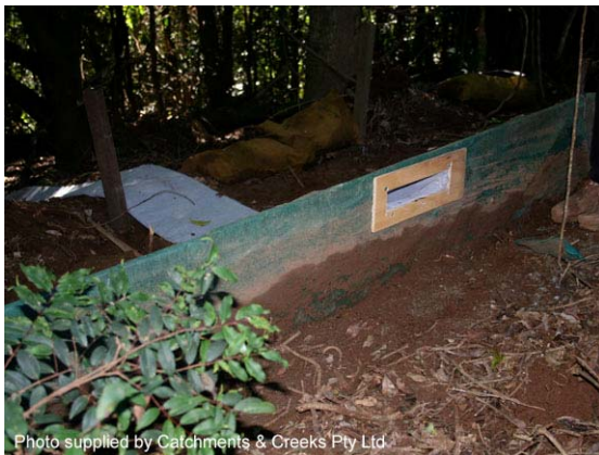
Photo 3 – Note filter tube inlet is raised above ground level to encourage ponding
