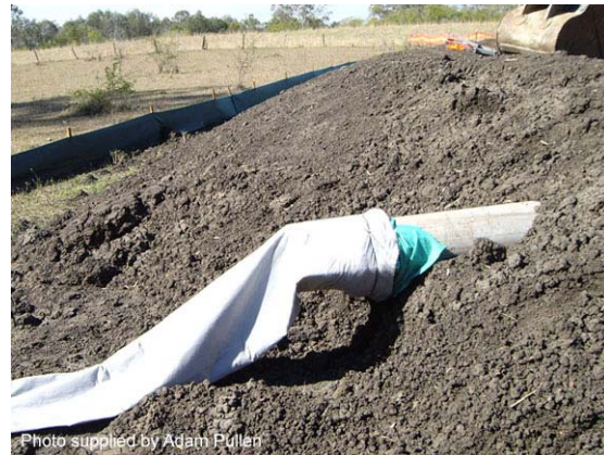
Photo 2 – Filter tube incorporated into a flow diversion bank
