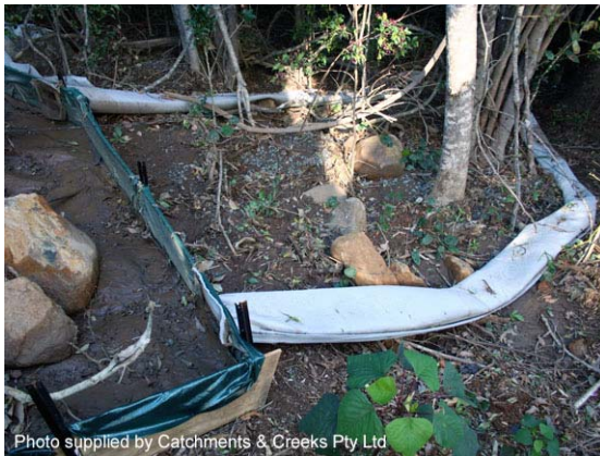
Photo 1 – Filter tube dam
