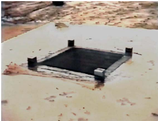
Photo 1 – Excavated drop inlet protection at top water level
