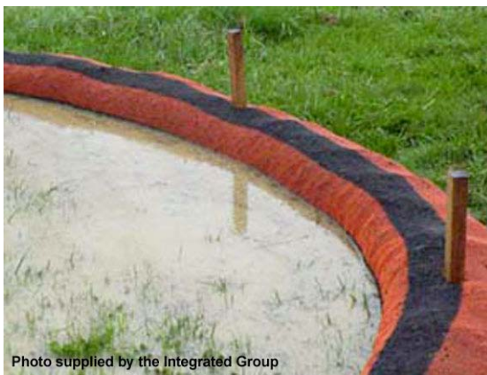
Photo 1 – Compost-filled sock being used to filter sheet flow
