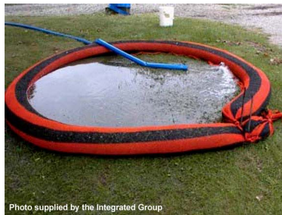
Photo 2 – Compost-filled sock being used during a de-watering activity
