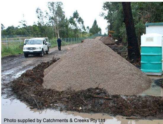
Photo 1 – Berm placed down-slope of a stockpile
