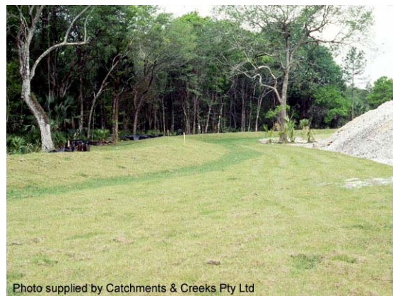
Photo 2 – Grassed buffer separating a stockpile from a grassed catch drain
