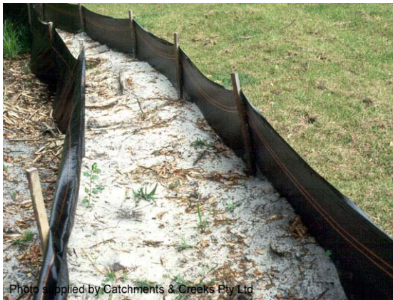
Incorporation of sediment fence with a buffer zone
