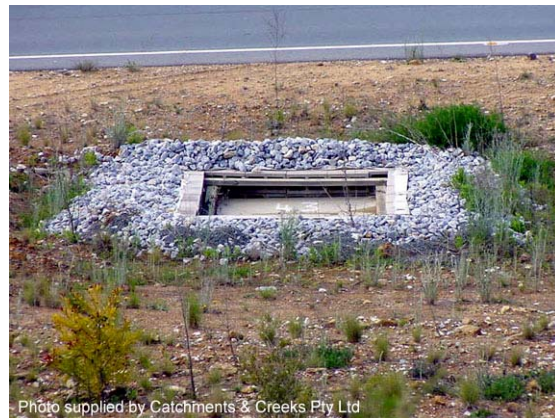
Photo 4 – Type B block and aggregate sediment trap (note, most blocks are turned sideways to allow through-flow)
