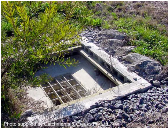
Photo 1 – Block and aggregate drop inlet protection supported by internal timber frame
