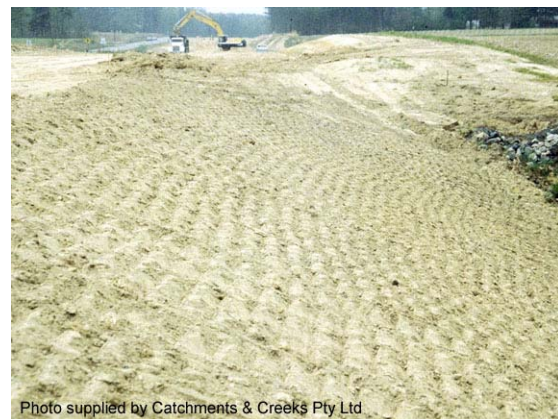
Photo 2 – Corrugated (roughened) surface
