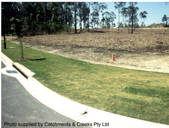
Photo 1 – Heavy mulching used for temporary erosion control measure instead of grassing (pre-building phase)
