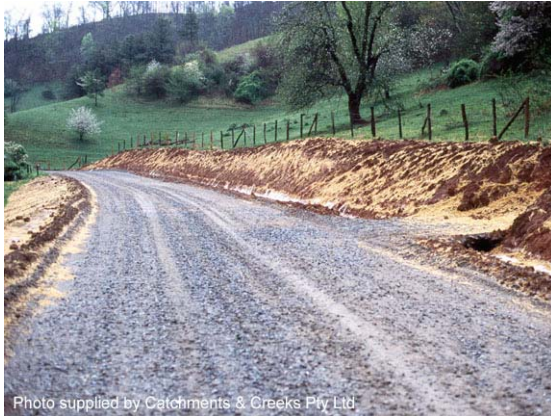
Photo 1 – Gravelling of construction access road
