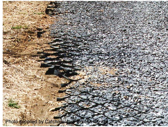
Photo 8 – Cellular confinement system
