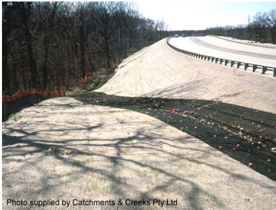
Photo 1 – Application of erosion control blankets and mats
