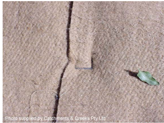
Photo 10 – Erosion control blanket
