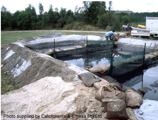
Photo 1 – Settling pond with internal baffles
