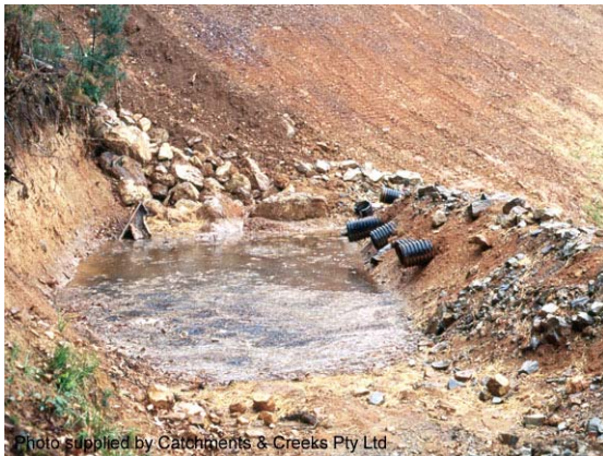
Photo 3 – Settling pond with siphon pipe overflow system
