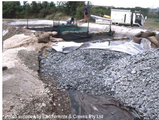
Photo 4 – Settling pond with rock spillway overflow system
