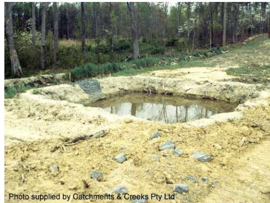
Photo 2 – Settling pond with rock filter dam outlet system
